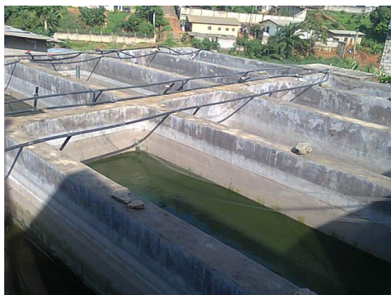
Plate 1 : Concrete fish ponds
